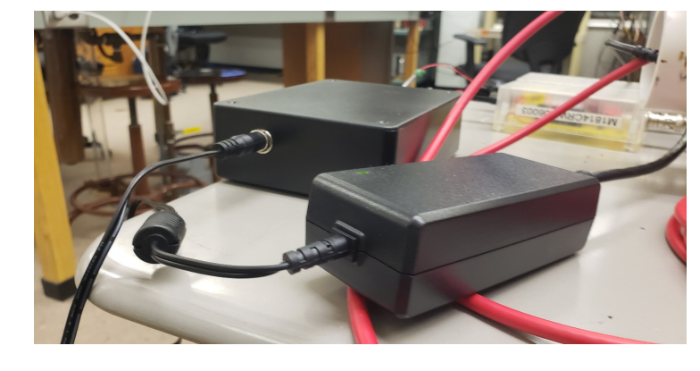
Laptop Charger plugged into the "Umbral Box" enclosure
