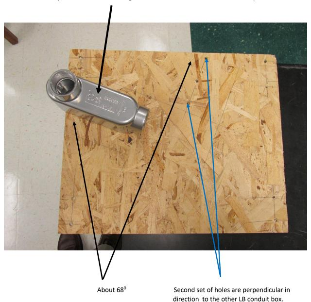
The counter over the LB conduit box should be the top counter in the stack, giving clearance for the cover.
